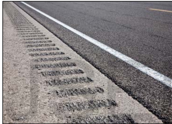
Figure 6. Continuous Milled-in Shoulder Rumble Strips (FHWA, 2017)
